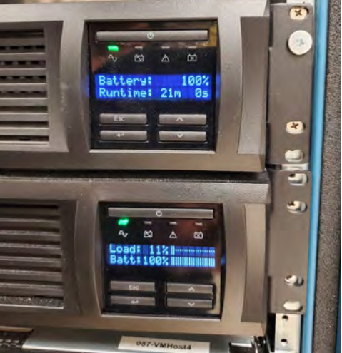
UPS units are rack mounted with no error or alarm messages displayed.
