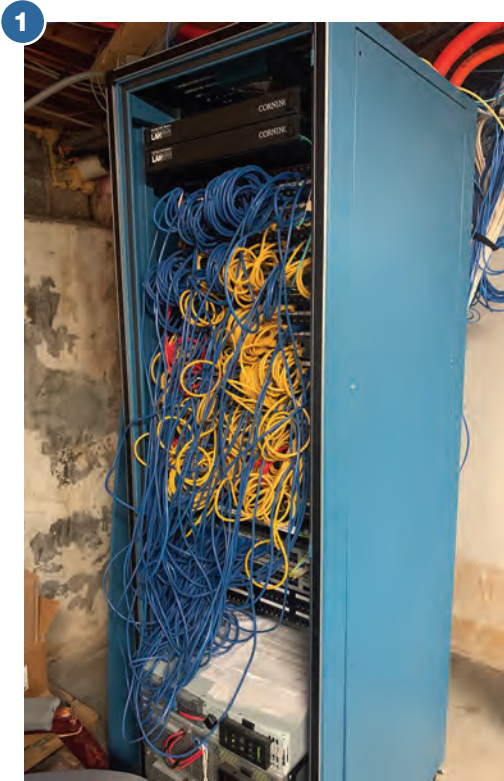
Photos, clockwise from top left: The open rack is in an unsecured area that is shared with custodial items. The space is below grade, a water pipe is installed directly over the rack, and cable management systems are lacking. Conduits are filled beyond capacities. There is a janitorial slop sink in the same space as the equipment.
