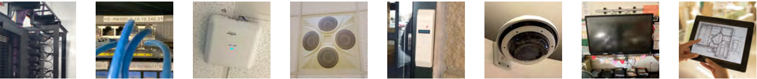
Building-based technology systems have evolved exponentially since wired telephone systems became common in the 1920s. Today’s technology systems are crucial to K12 daily operations. Critical components include (above left to right) Telecom Rooms, wired and wireless network equipment, Public Address, Access Control, Video Surveillance, classroom displays, and student devices.
