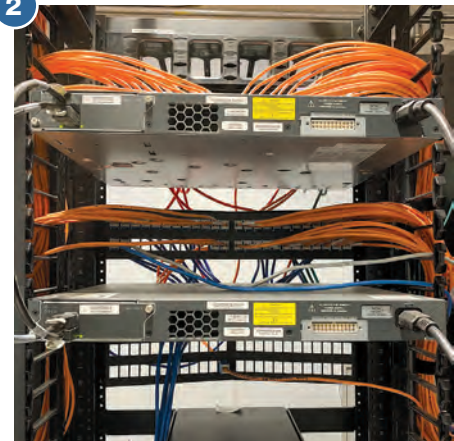
Photos, clockwise from top left: The dedicated secure space includes (3) newer equipment racks. The racks include properly installed cable lengths and management. A properly labeled electrical outlet from the building's emergency generator. A properly installed grounding bar with all components correctly connected.
