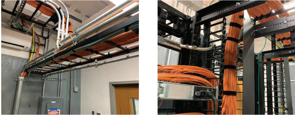
Cable management systems in a TR should accommodate both overhead (right) and vertical (far right) cables.
