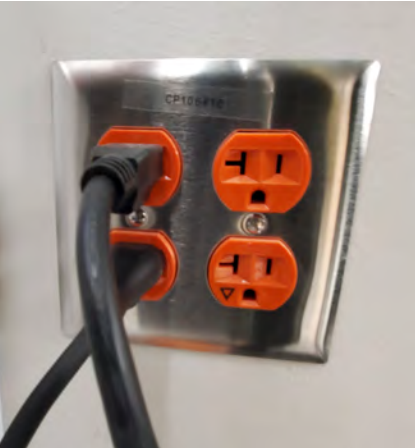
A dedicated electrical circuit with (2) 20A outlets (left) and an emergency generator outlet with proper labeling.
