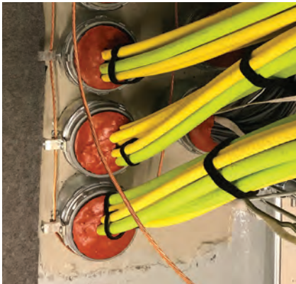
Conduit with proper fill ratio and properly installed firestop. Photo©BICSI. All rights acknowledged.
