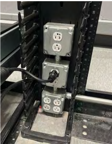
Electrical outlets should be mounted to all racks.
